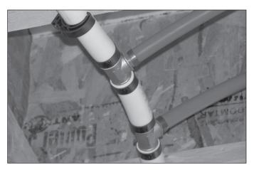
Zurn PEX large diameter tube and tee fittings shown in trunk and branch method.
