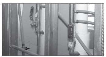
Zurn PEX tubing connected to copper manifolds using copper crimp rings.
