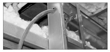
Zurn PEX tubing sleeved through steel stud for protection.
