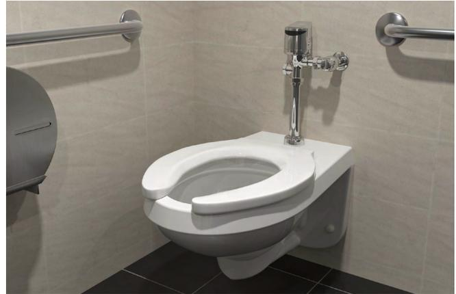
When it comes to lasting performance, this flush valve collection rises above the rest. Its winning combination of gear-driven ceramic cartridge operation and thermoplastic elastomer (TPE) diaphragm delivers superior reliability and outperforms solenoid-operated models.
