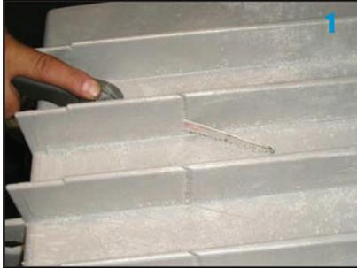
1. Place outlet onto catch basin in required location. Mark top and bottom of outlet onto ribs. Cut ribs with handsaw.
