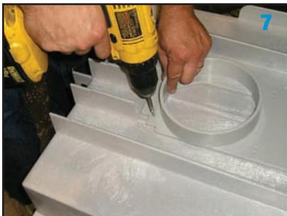
7. Once outlet is placed, attach outlet with supplied screws.
