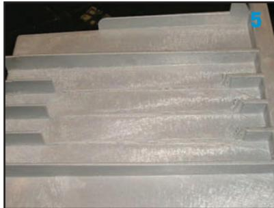
5. Rough fit out onto basin, ensuring there are no obstructions and outlet seats flush.
