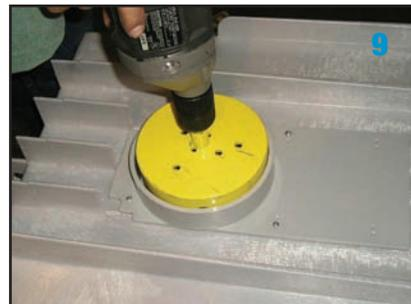
9. Once outlet is firmly secure, drill outlet/catch basin hole with a hole saw.
