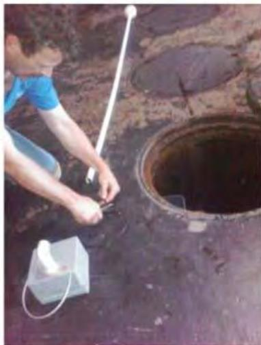
At top end of PVC pipe, cut black wire approximately 6" longer than PVC pipe. Strip black wire shielding to expose wires but do not strip individual wire jacketing.
