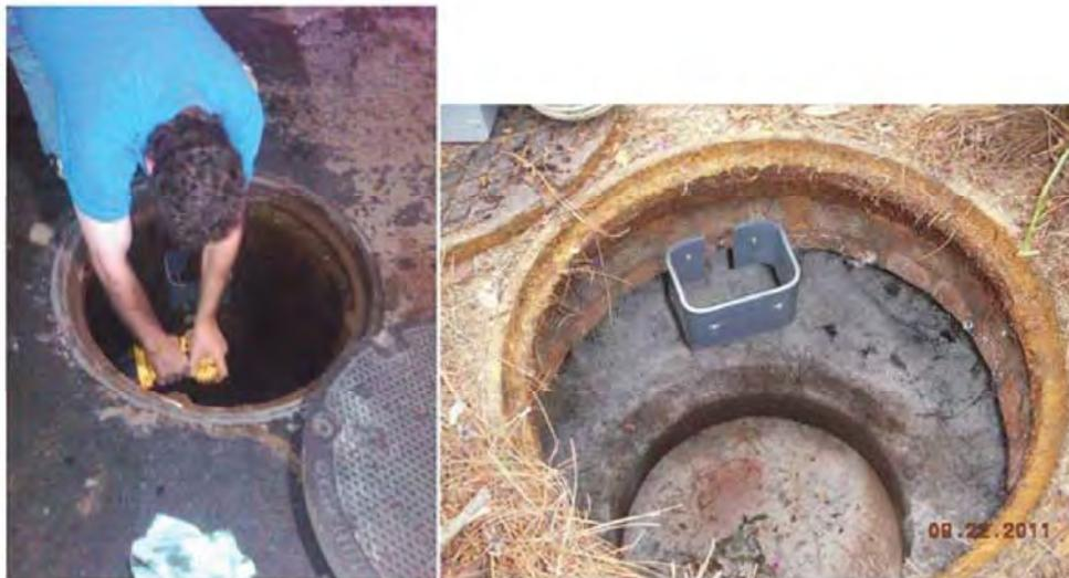
Install U-bracket level in manway riser with 2 mounting bolts provided. Bolt holes should be drilled into the riser approximately 15" from grade in a position where underwater probe does not have obstructions and the manway cover will not interfere or damage the control box.
