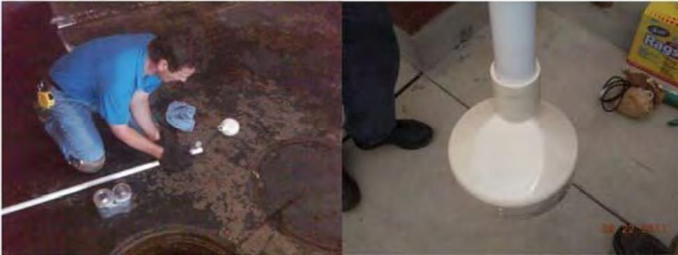
Cut ¾" PVC pipe to length (**A** + ½ **B**) so probe end is positioned in the middle of the interceptor liquid level. Run the black wire from the probe through the PVC pipe. Secure probe to the PVC pipe with PVC cement to create a waterproof seal.
