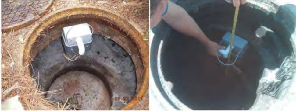
Insert control box into the U-bracket as shown. Measure the distance from the ¾" PVC elbow (with 6 wires) to the top of the grease layer/liquid level (Dimension **A**). Then measure the liquid level to the bottom of the tank (Dimension **B**) [See Figure 1]. Tank bottom must have no sediment build-up to insure accurate measurement.
