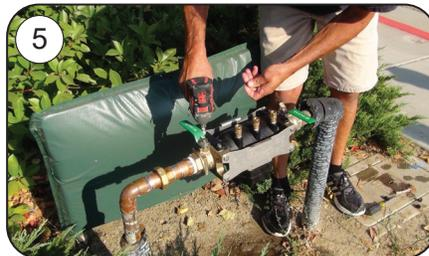
5 Remove Flush Fitting Tool and reinstall EZSwap™ Pressure Vessel.
