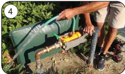
4 Turn on inlet ball valve, direct water to landscaping or safe drain, and flush until clear.
