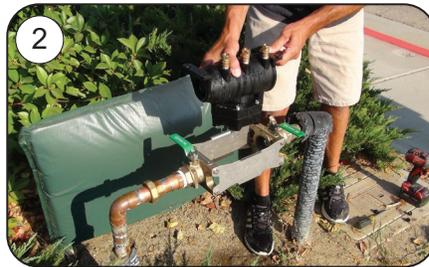
2 Un-bolt and remove EZSwap™ Pressure Vessel.
