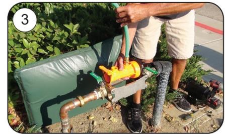
3 Drop in and install Flush Fitting Tool. Attach hose.
